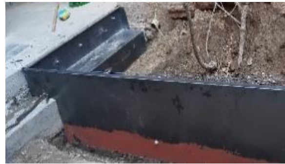
Figure 25: Installing the steel edges of the stairs. [Source: Researchers]
