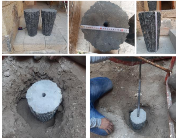
Figure 23: Basalt bases during the implementation [Source: Researchers]
