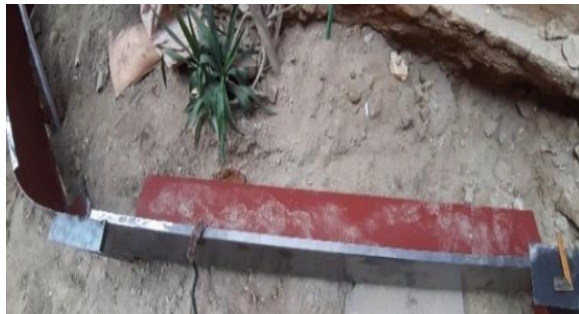
Figure 27: Detailed drawing for the bent steel column and planted area steel edges and how they had installed with the reference to the underground tunnel, second photo for the bent steel edges during its implementation. [Source: Researchers]
