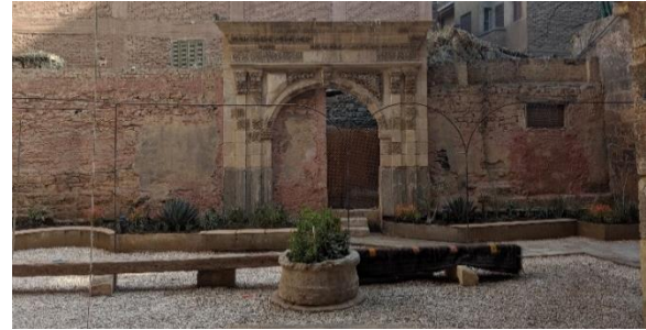
Figure 17: the new entrance for the background area within the historical gate, stairs after repositioned the door. [Source: Researchers]
