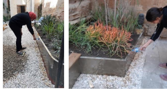
Figure 20: Spraying water to accelerate rusting. [Source: Researchers]
