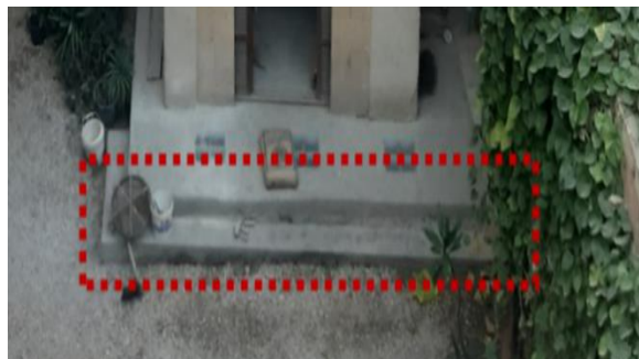
Figure 24: The preexisting stairs before installing the al-Bustan. [Source: Researchers]
