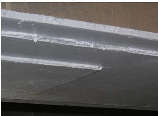
**Fig. 2** Adding Plates Welded to Lower Flange of the Tested Bridge
