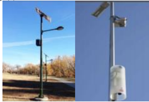
Fig. 9 - Off-grid light fixtures and digital addition to LED fixtures
