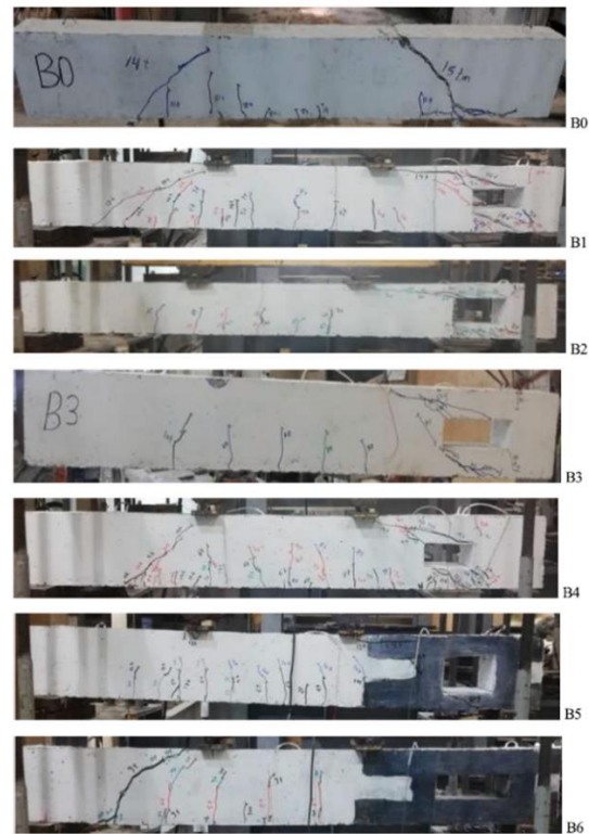
Figure 16: Crack patterns and failure modes [40]
